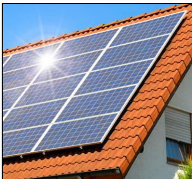
Figure 2: RMPV (mounted panels)
