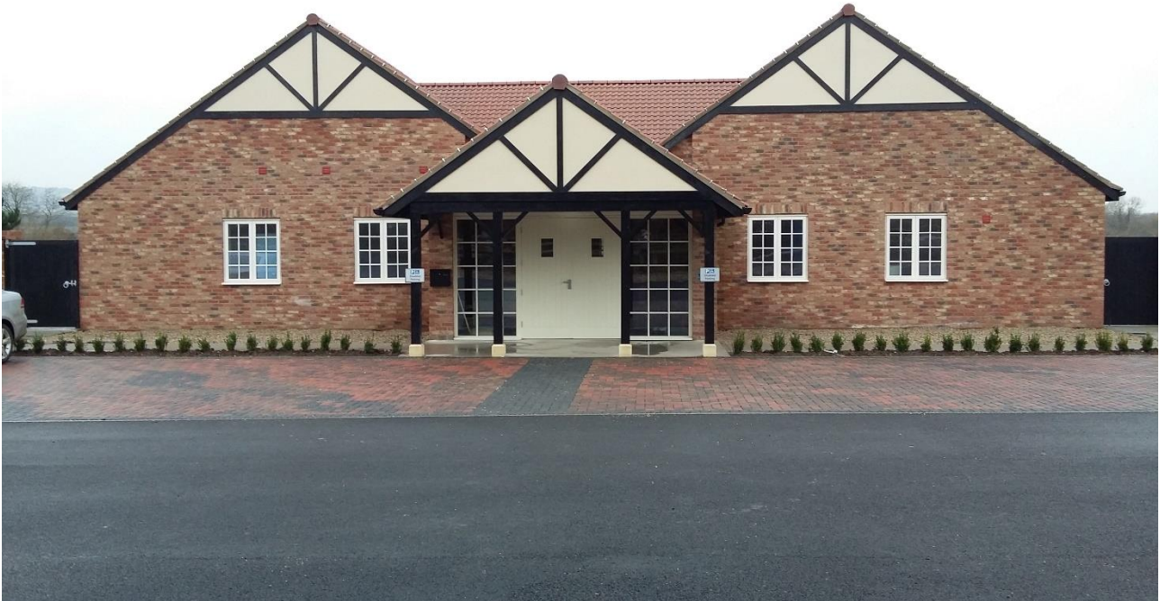
Figure 67: Wintringham Village Hall (east elevation)
