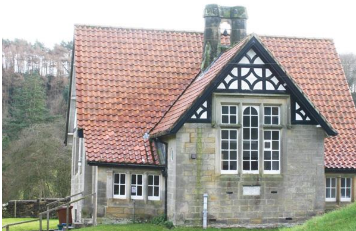
Figure 35: Darley Memorial Hall - Lastingham and Spaunton
