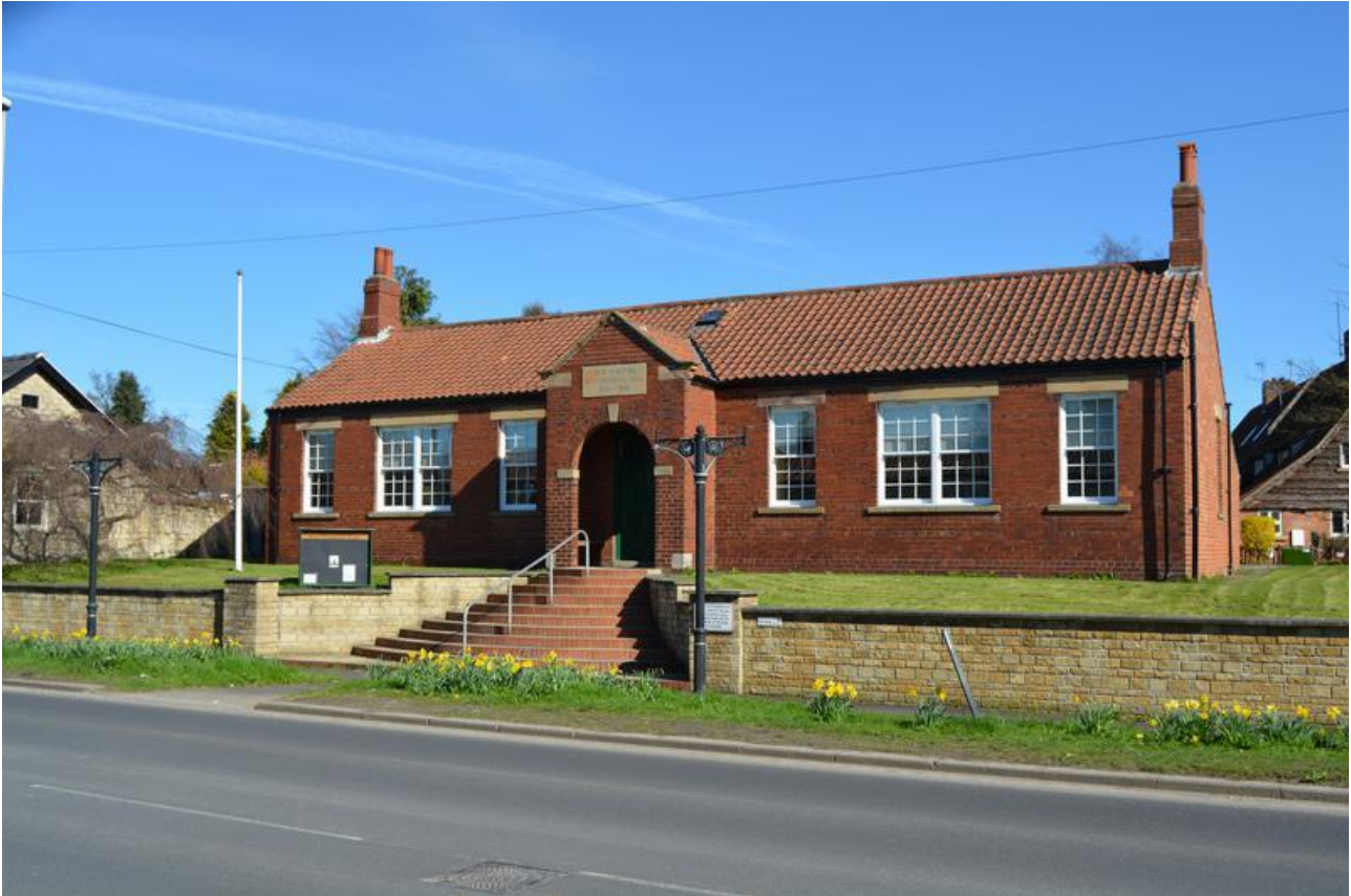
Figure 44: Old Malton Village Hall
