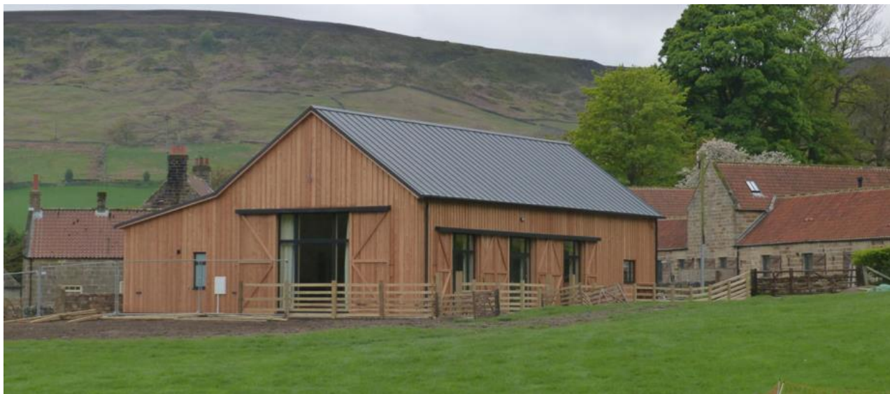
Figure 22: Farndale Village Hall
