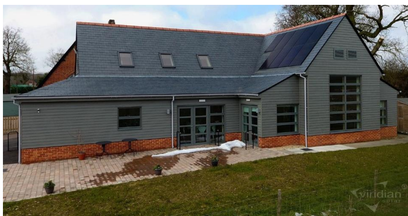
Figure 4: In-roof PV example from Viridian Solar
